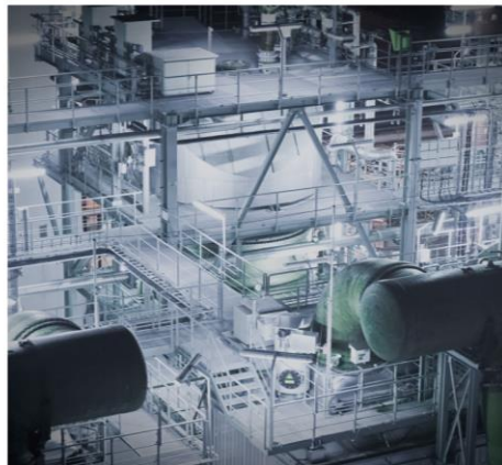
Power Monitoring and Control System
