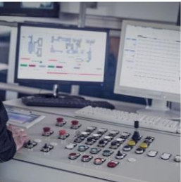
Heating, Ventilating, and Air Conditioning System
