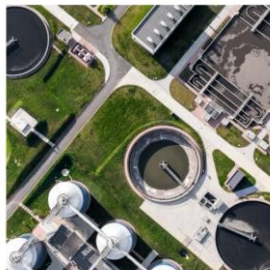
Water Supply Facility Management System
