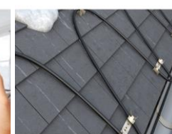
ROOF AND GUTTER DE-ICING
